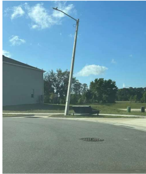
Leaning Lightpole at SW Bend of Laurent Loop
