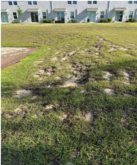
Pond 300 Eastern Bank Erosion
