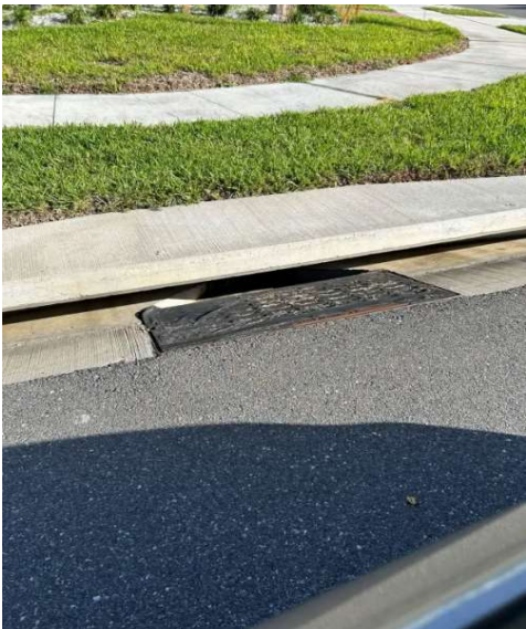
Inlet with filter fabric in Phase 3
