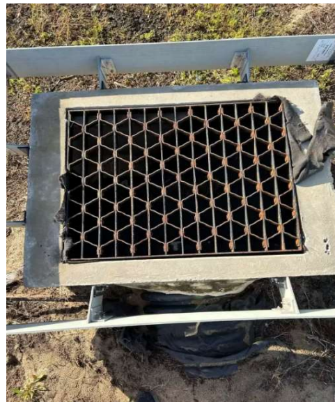
CS-80 with filter fabric still present under grate
