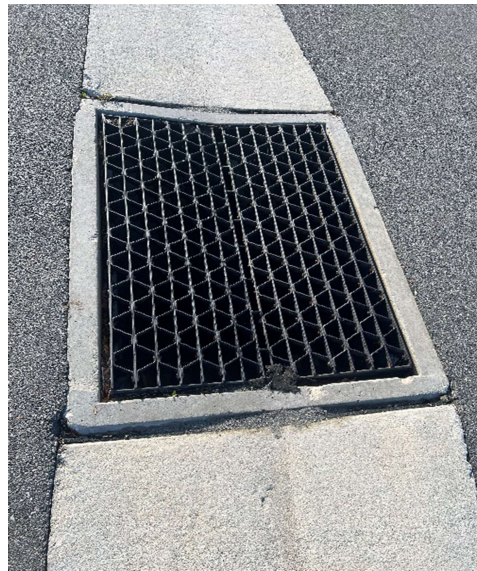
V-Inlet w/ Filter Fabric
