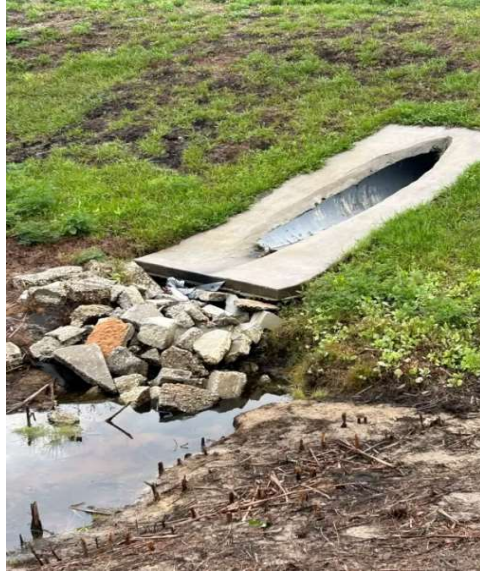
Pond 300 Mitered End Section
